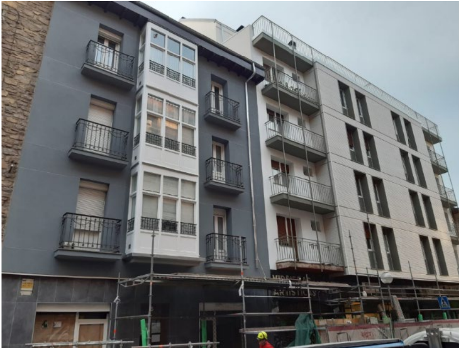
Retrofitted building Aldabe 5 in demo district Coronación. Credits@Vitoria-Gasteiz
