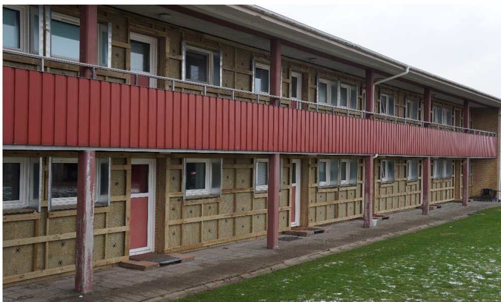
Figure 13: B42 Department 13. New facade insulation under construction in 2018
