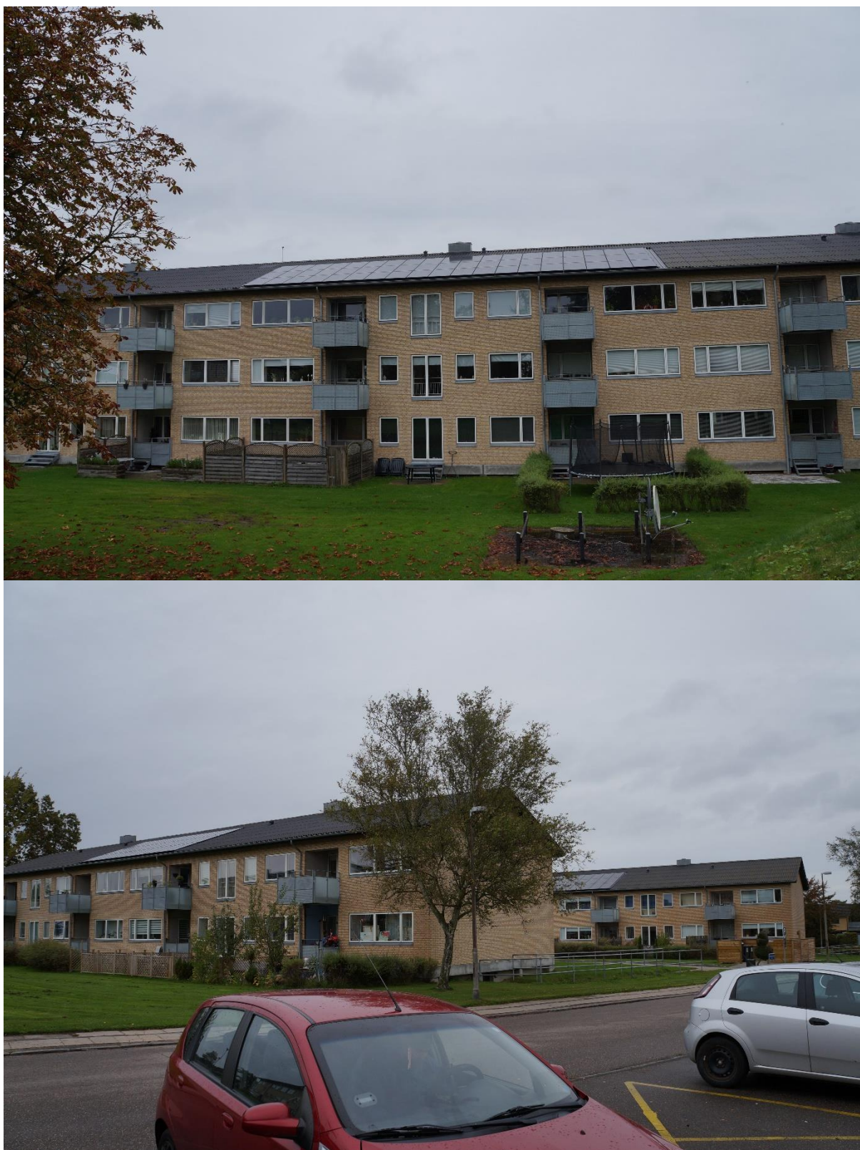
Figure 7: SAB Department 22 with building integrated solar cells, in total on 19 buildings.
