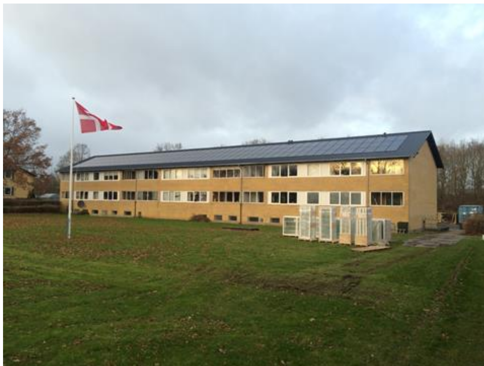
Figure 3: SOBO Department 11: Building integrated solar cells.
