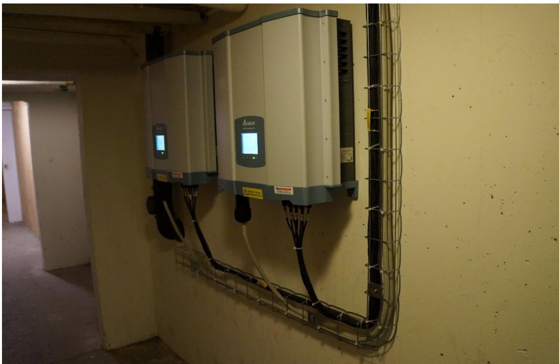
Figure 21: SAB Department 22: Inverters for solar cell systems.
