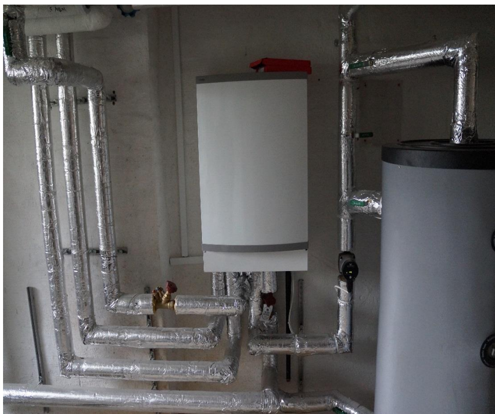
Figure 4: SOBO Department 11: New heat exchanger for district heating.
