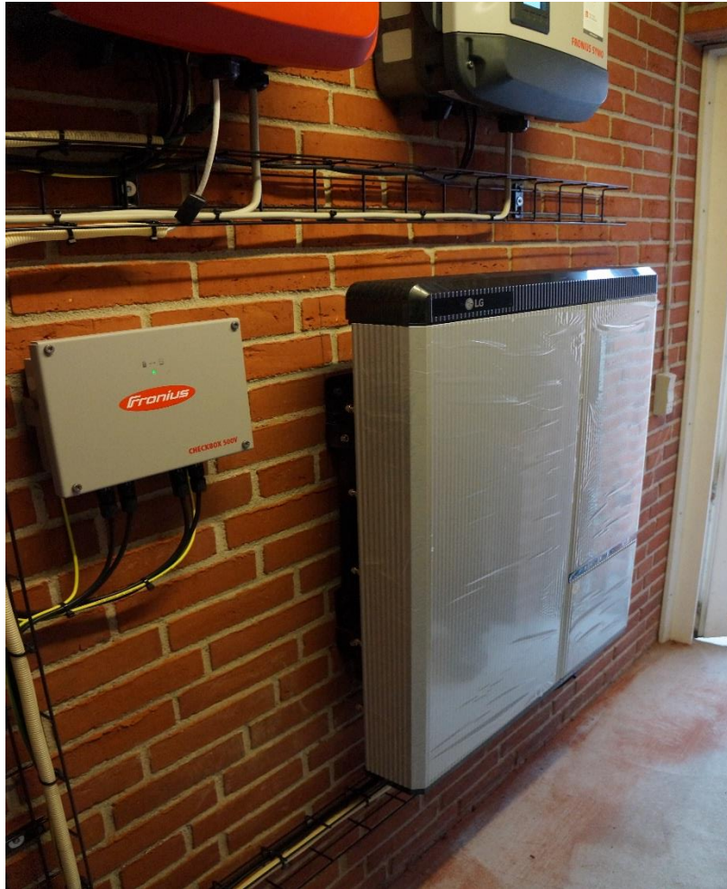
Figure 17: B42 Department 21: Battery solution in combination with solar cells.
