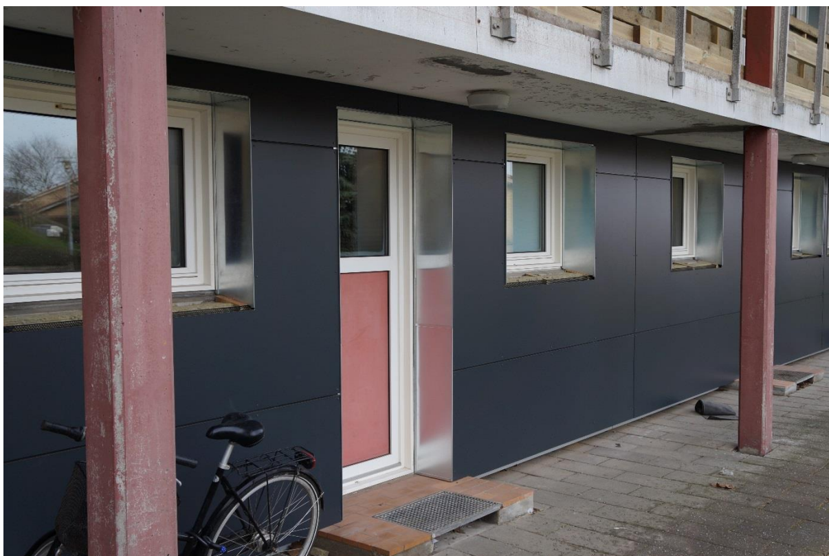
Figure 24: B42 Department 13: New facade insulation.
