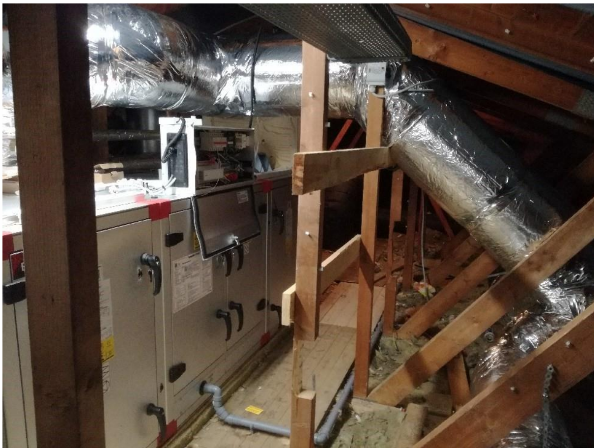
Figure 23: B42 Department 21: New ventilation systems with heat recovery.
