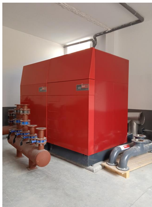
Figure 11: Gas boiler
